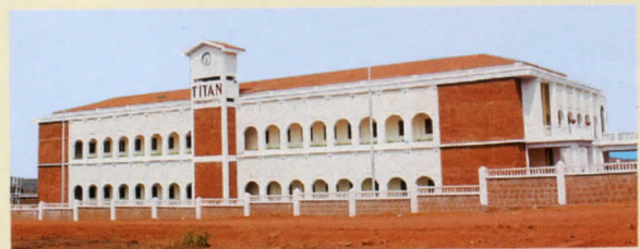
The electronic circuit plant of Titan Time Products, Goa.
