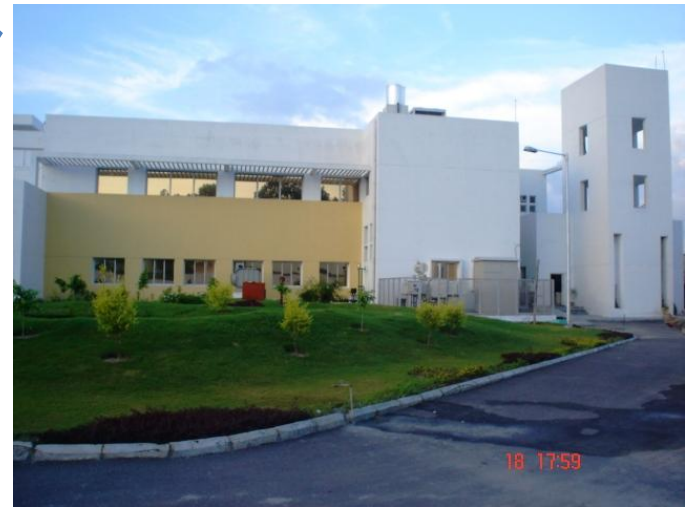
Dehradun Assembly Plant
